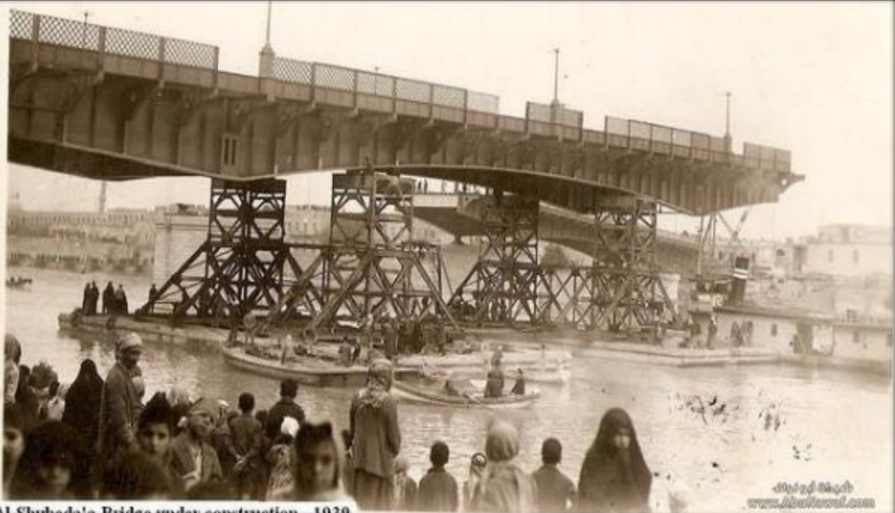
Al-Shuhada's Bridge under construction - 1939
